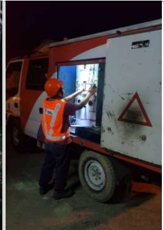
b) Fault locate test set in a lorry.
