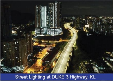
Street Lighting at DUKE 3 Highway, KL
