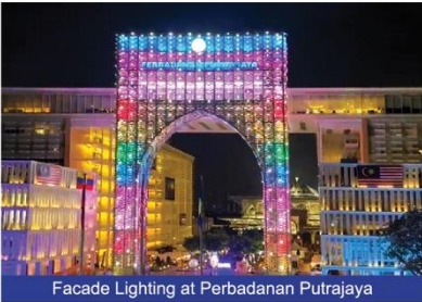
Facade Lighting at Perbadanan Putrajaya
